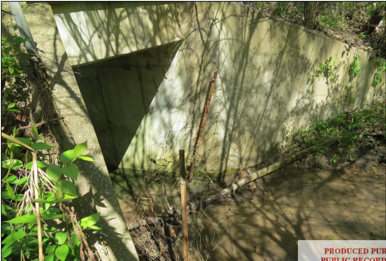
RIGHT SIDE VIEW OF BRIDGE (INLET)
